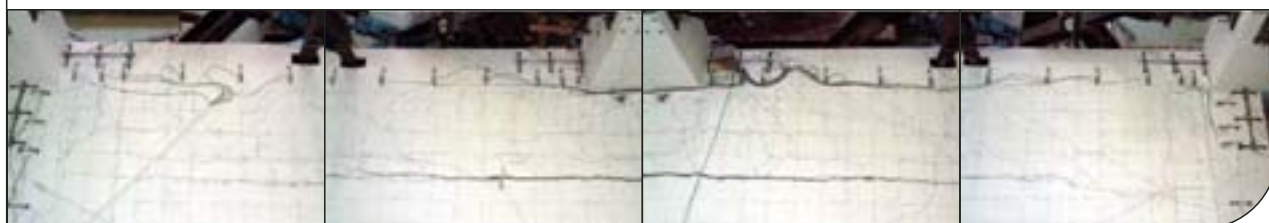
Figure 1 Separation of floor slab putting high strains on topping reinforcement. Source: University of Canterbury Civil Engineering Department, J Matthews
