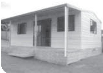
Figure 2: A unit in its final position
